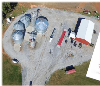
Aerial of ASR Grain Facilities
